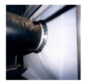
Penetrations can be accommodated and sealed up to 500mm in diameter.
