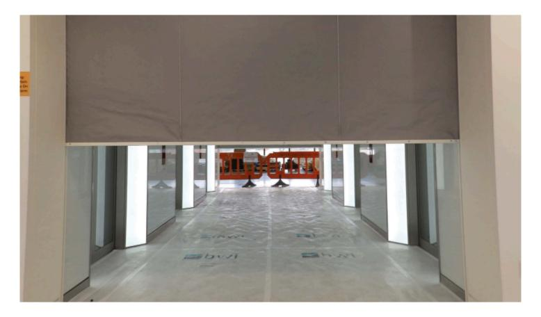
Despite BLE Smoke & Fire Curtains continual raising of the performance bar with their 240 minute integrity fire curtain, it is recognised that not all buildings require this level of protection. Therefore BLE introduced the FC1; a 60-minute integrity solution built with all the same build quality and options as the FC2.
